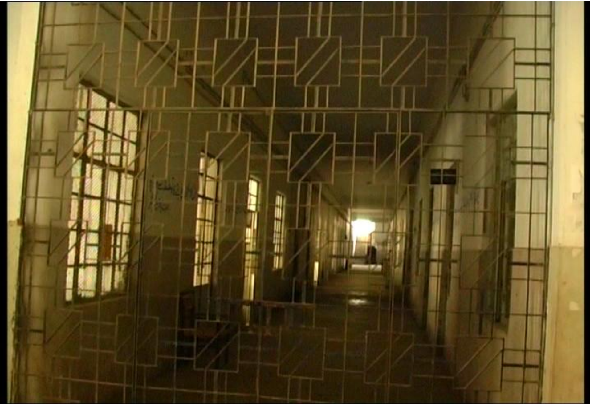
School Corridor (Before)
