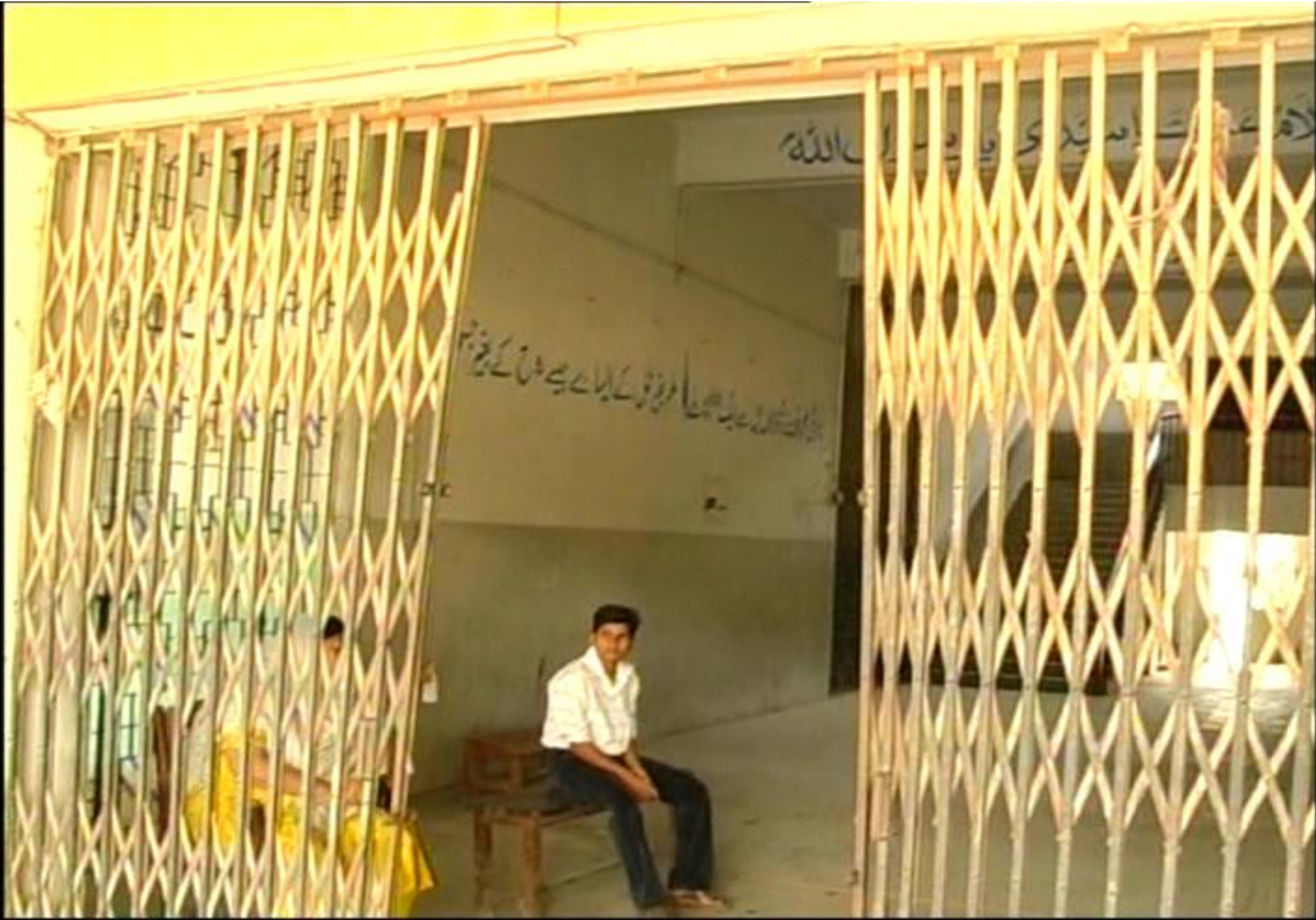
Front Part of Entrance (Before)
