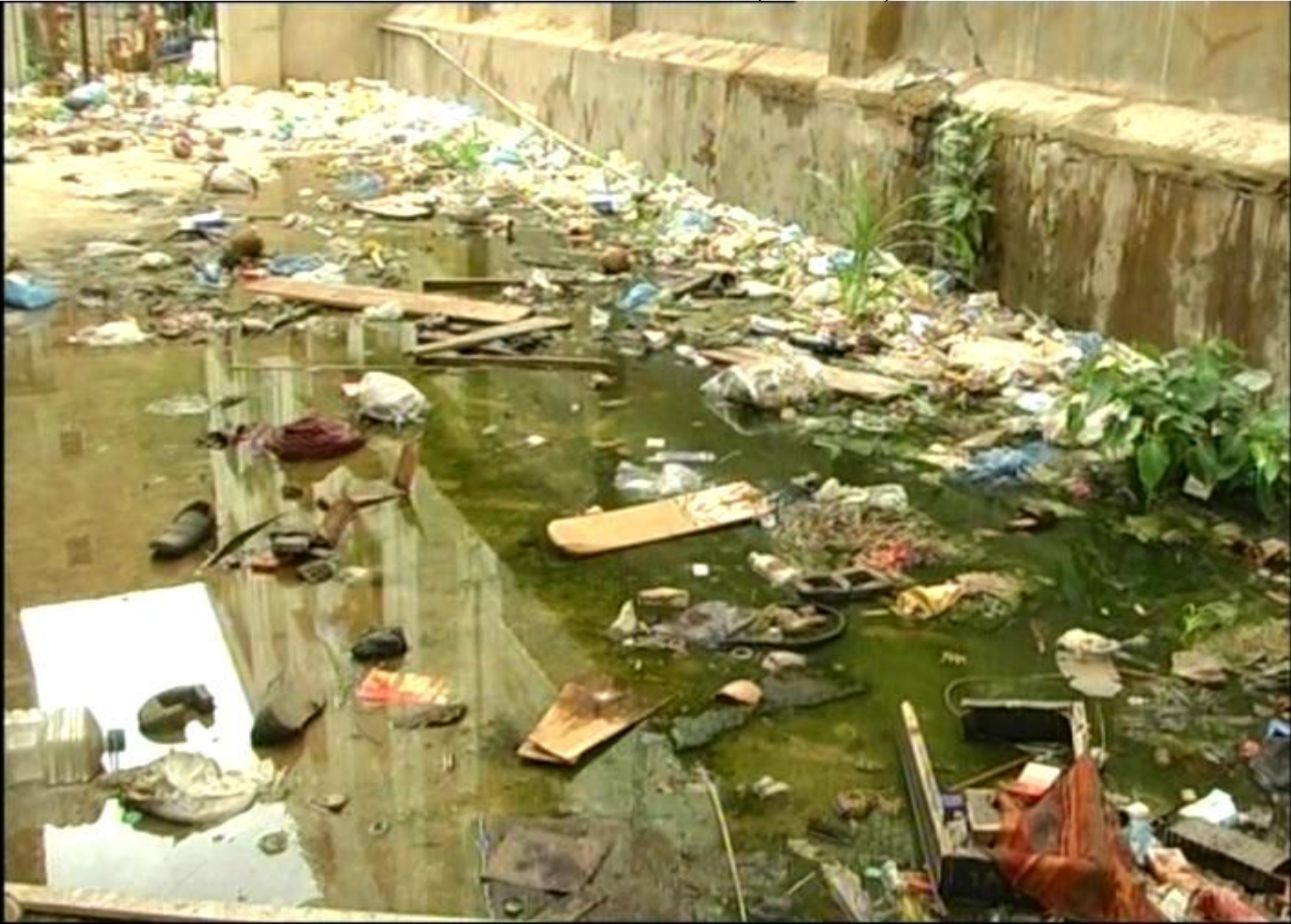
Backside of School (Before)
